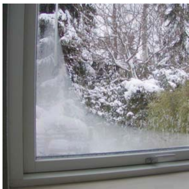
Figure 6: Window water condensation is often sign of poor ventilation in dwellings; Right: Prevalence and odds ratio for rhinitis among children versus condensation on windows pane in bedroom [11]
